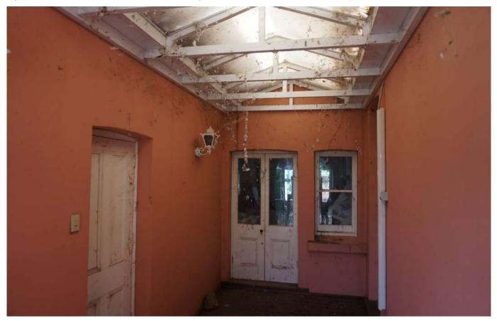
Figure 18. Covered vestibule connecting the central and western wings of the house noting wall beyond proposed for removal (Element Advisory, 2023)
