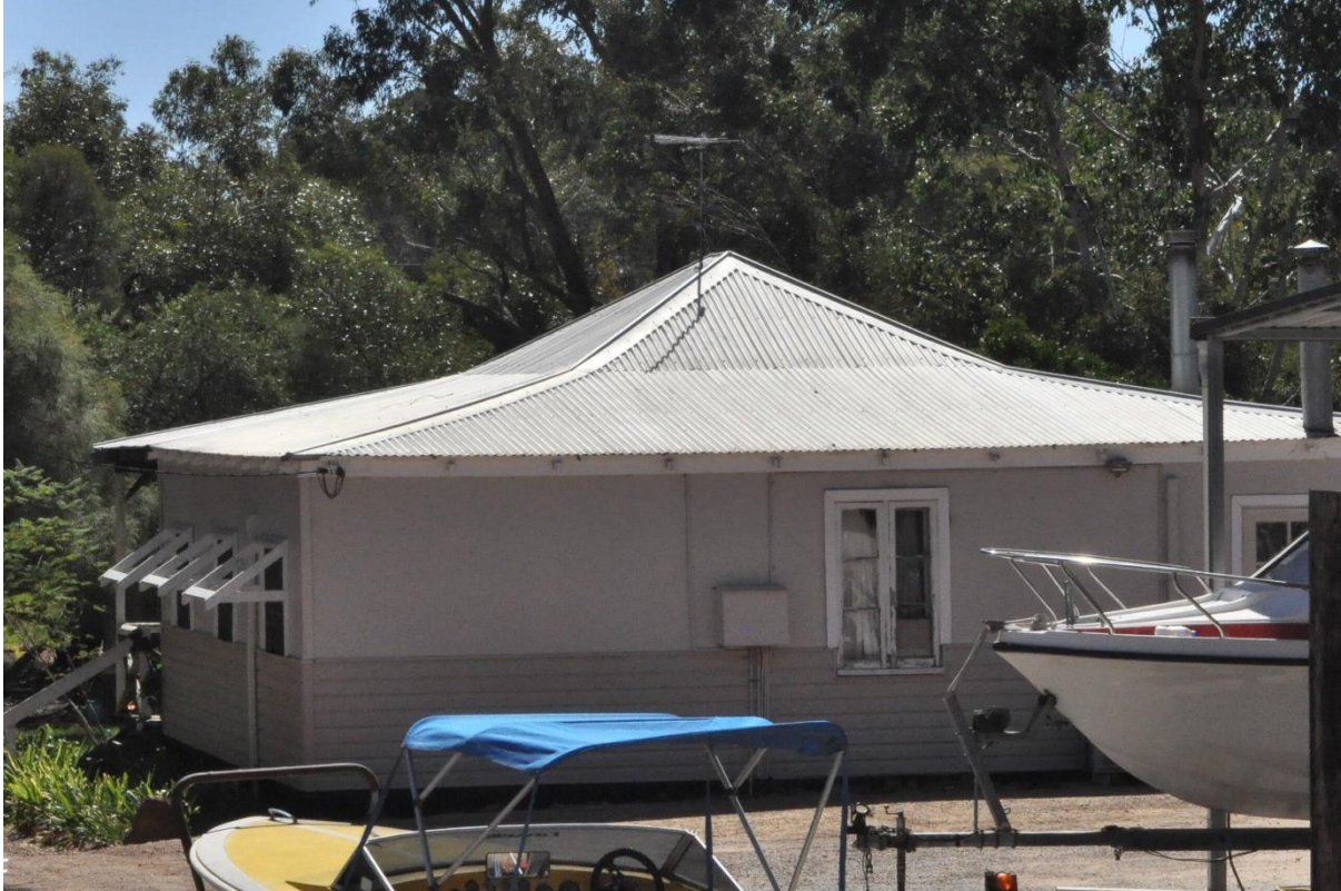
View of South Elevation, 10 April 2024. Source Shire of Mundaring
