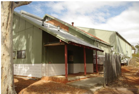
Side view showing addition to the original school building.
