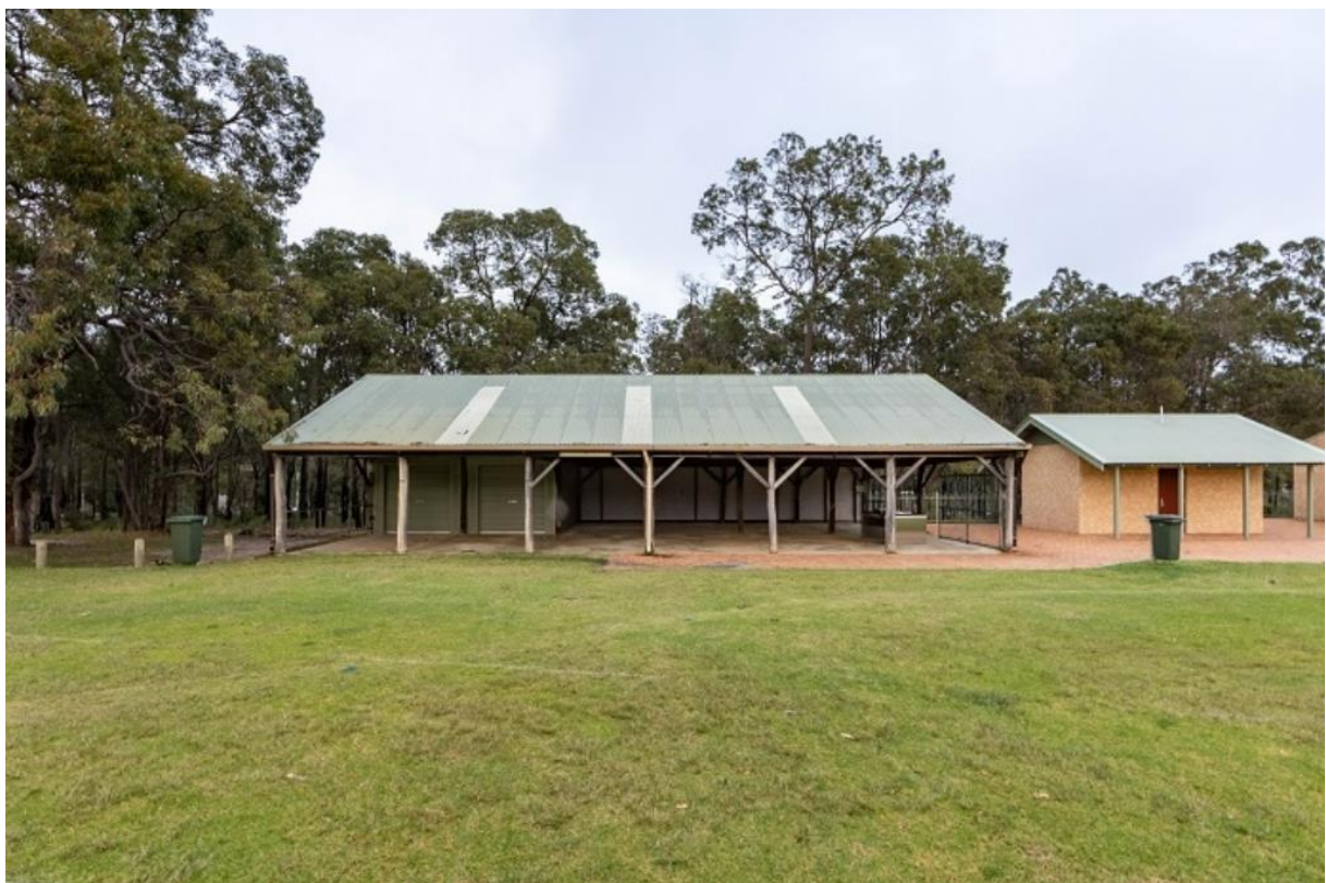
North-east elevation, 2020 (Source: Shire of Mundaring)
