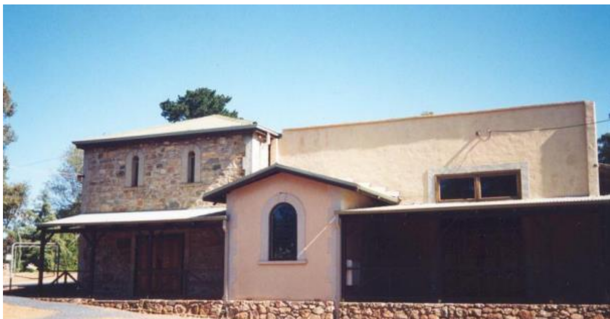
Darlington Hall: Front (north-east) elevation, August 1995 (Source: Bruce Callow and Associates Pty Ltd)
