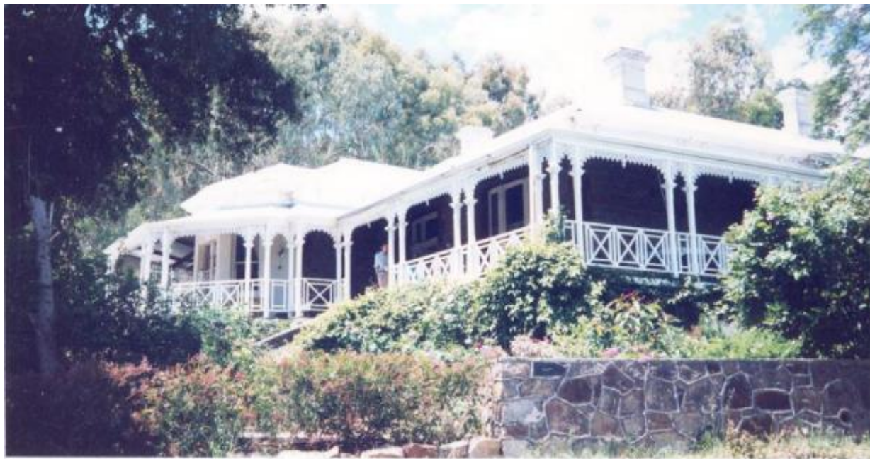
Front, south-west elevation, November 1995 (Source: Bruce Callow and Associates Pty Ltd)
