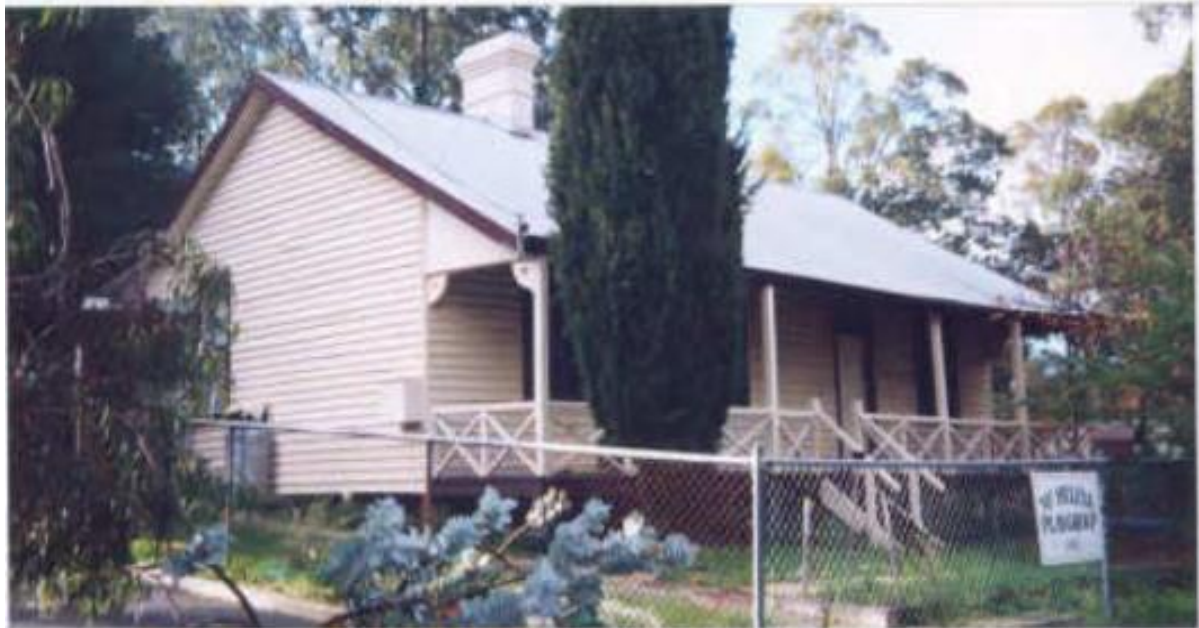
Front elevation, July 1995 (Source: Bruce Callow and Associates Pty Ltd)
