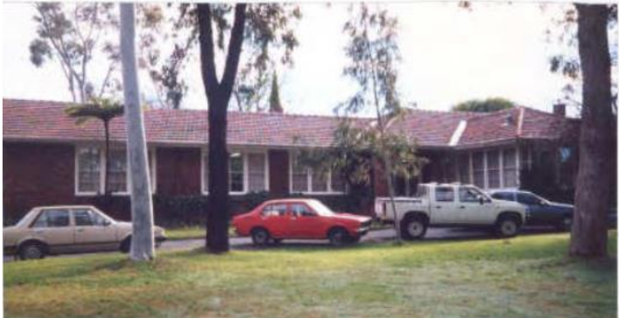
Original Administration building, July 1995 (Source: Bruce Callow and Associates Pty Ltd)
