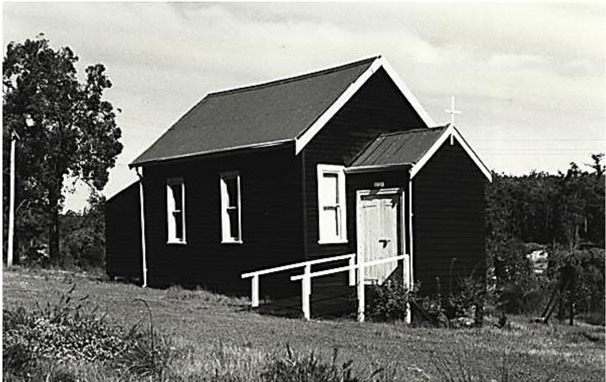
Front elevation of the church (date 1981)
