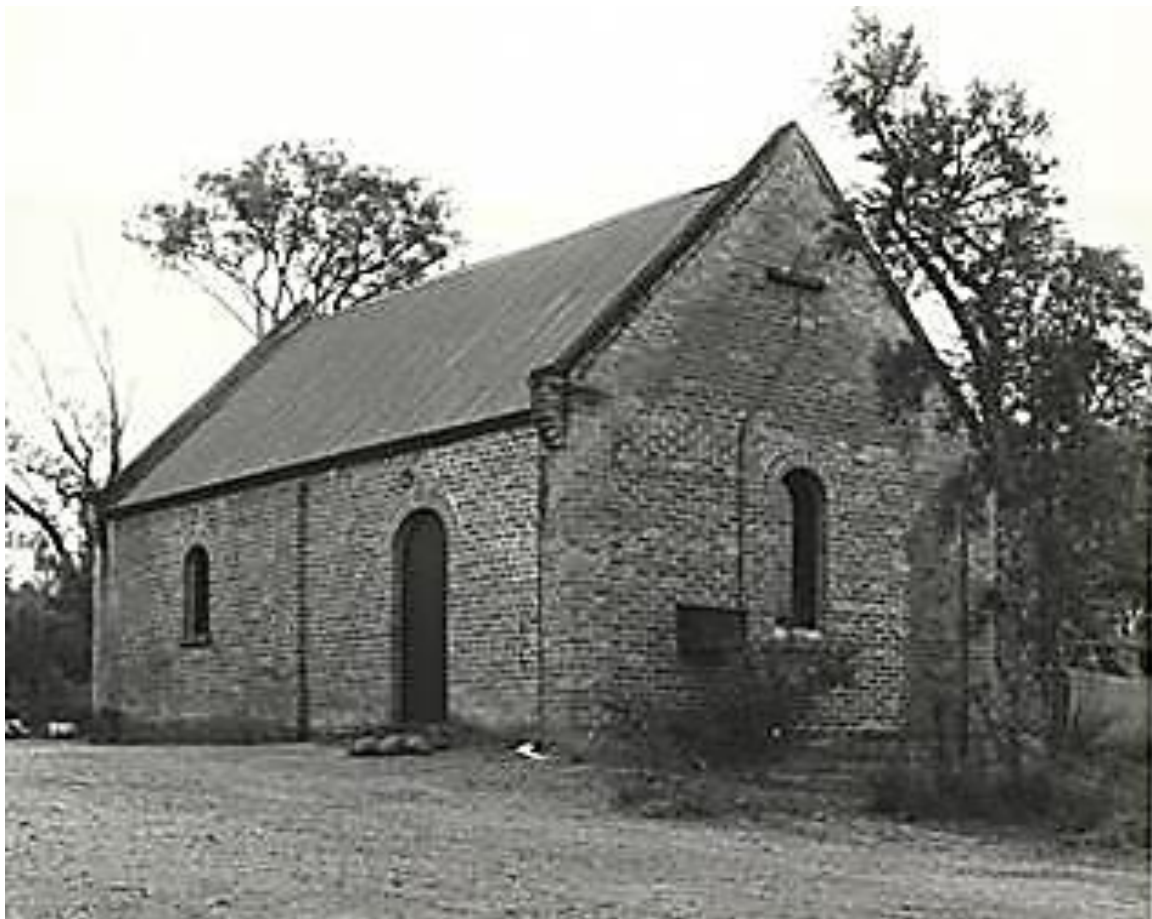
Left corner elevation of church (date unknown) (Source: Heritage Council of Western Australia, photo taken by F.A. Sharr)
