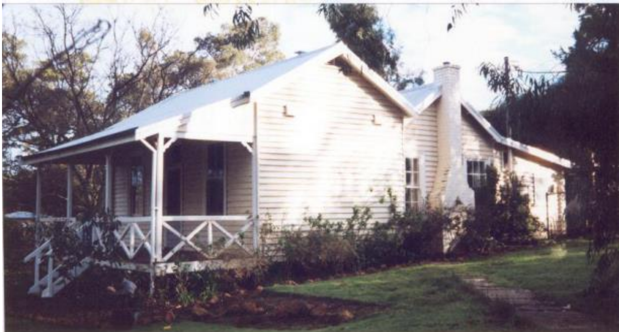
Old School House Sawyers Valley - looking from east, July 1995. (Source: Bruce Callow and Associates Pty Ltd)
