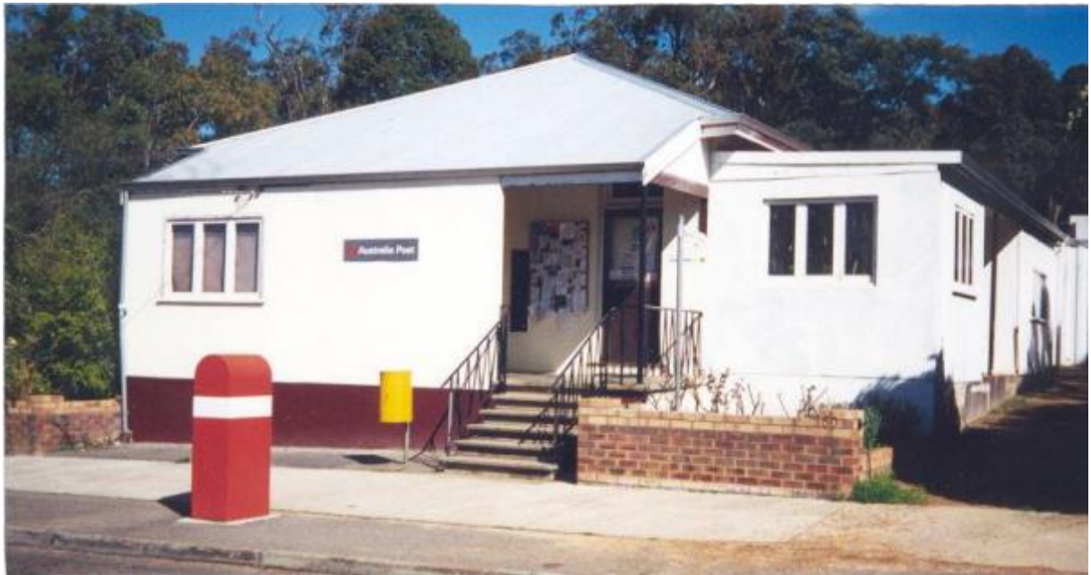
Front, eastern elevation, August 1995 (Source: Bruce Callow and Associates Pty Ltd)
