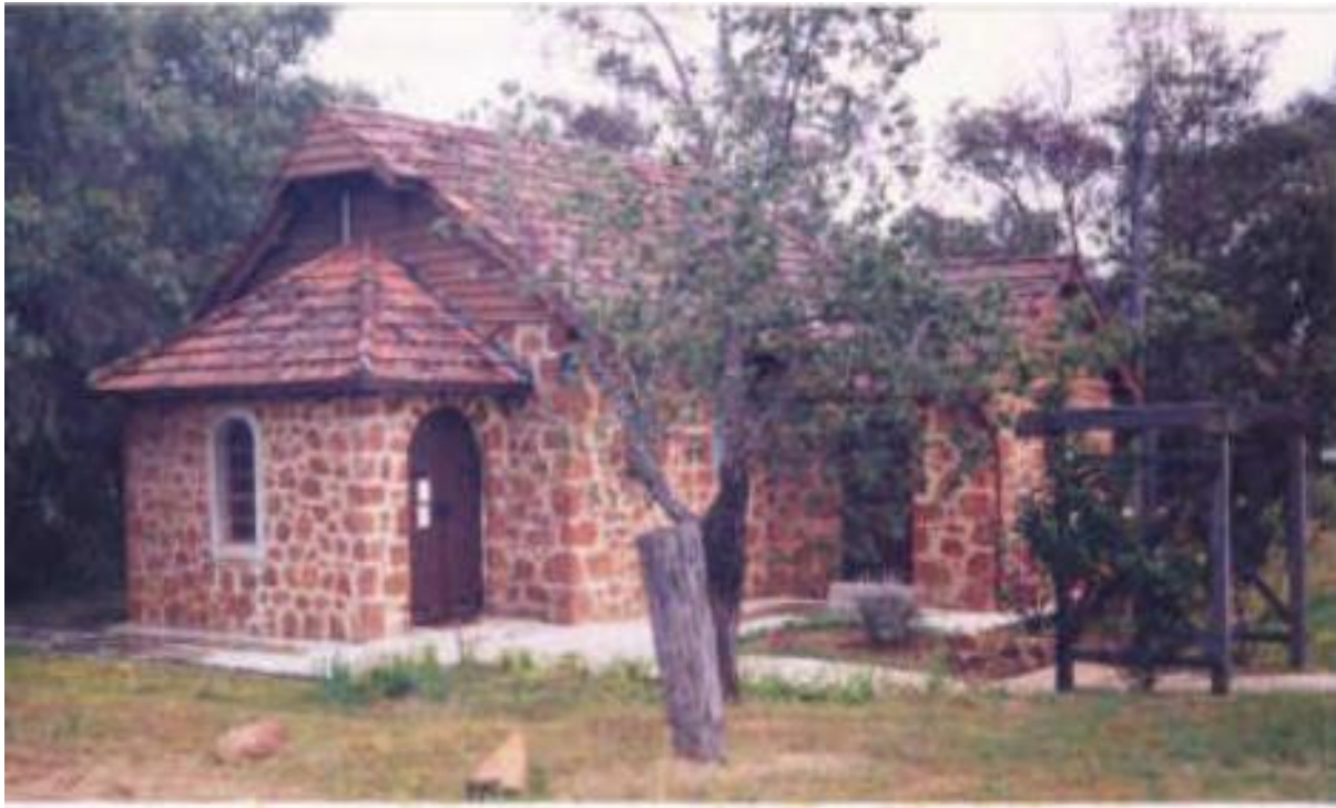
Front elevation, showing entry porch, October 1995 (Source: Bruce Callow and Associates Pty Ltd)
