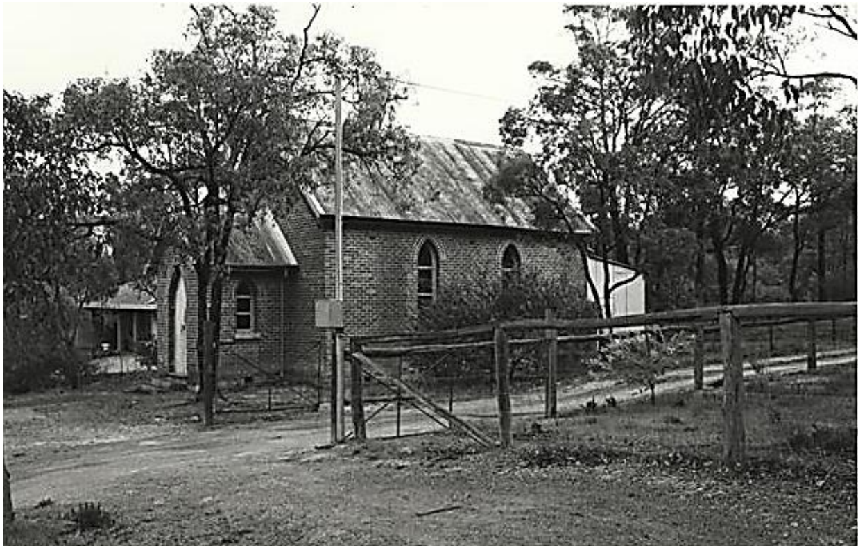
Right side elevation of the church (Source: Heritage Council of Western Australia, photo taken by F.A. Sharr)
