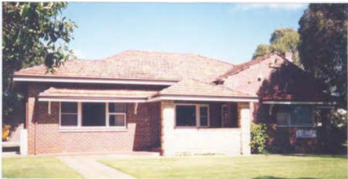
North elevation of 'Old' Shire Secretary's House, 1982/1983 (Source: Bruce Callow and Associates Pty Ltd)
