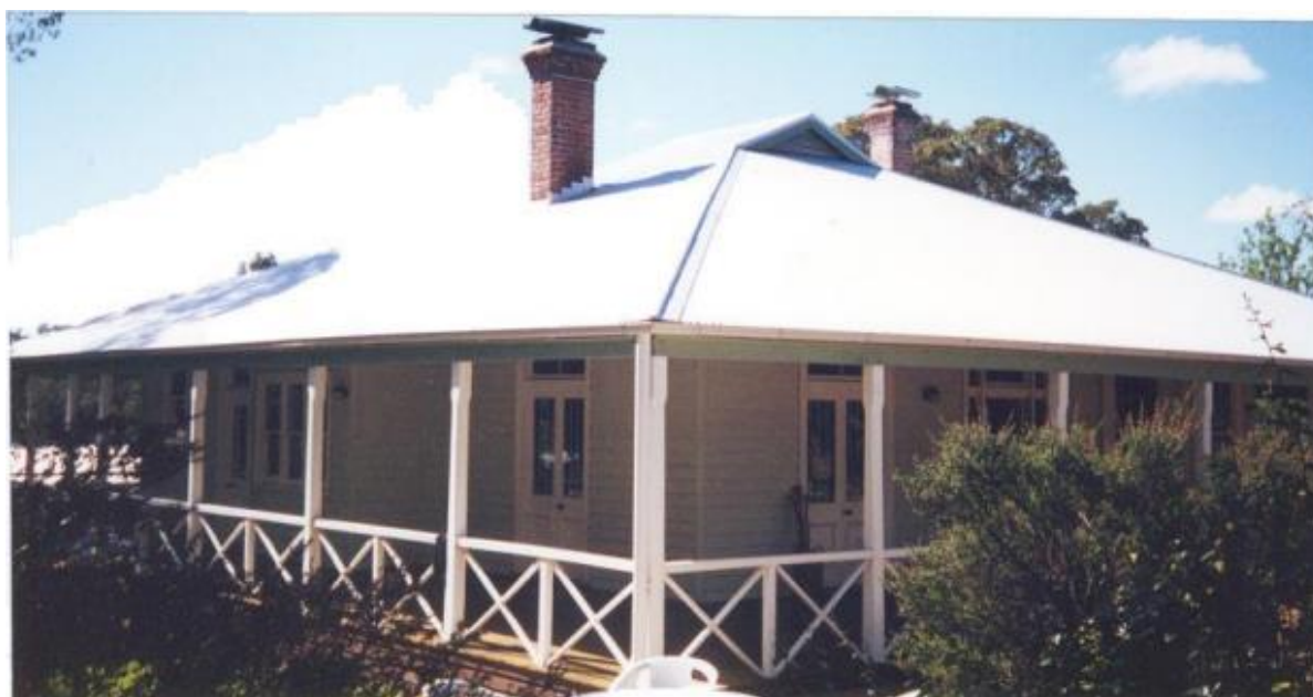
South-West elevations, August 1995 (Source: Bruce Callow and Associates Pty Ltd)
