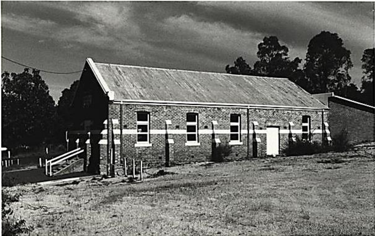
Right side elevation of the building (October 1981) (Source: Heritage Council of Western Australia, photo taken by F.A. Sharr)
