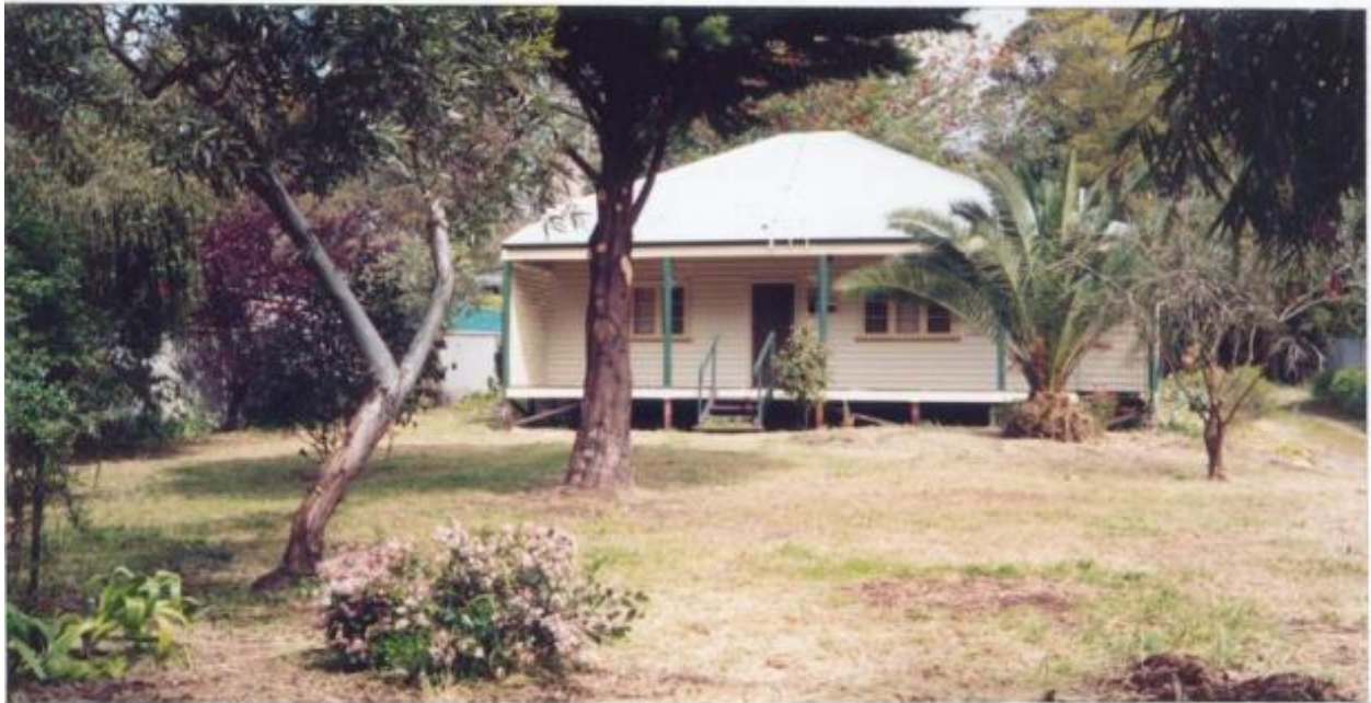
East elevation, October 1995 (Source: Bruce Callow and Associates Pty Ltd)
