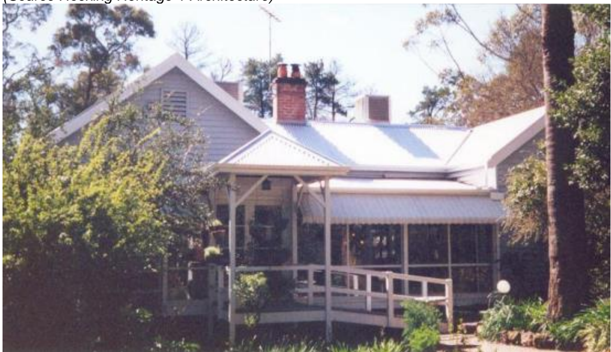
South elevation, , August 1995 (Source: Bruce Callow and Associates Pty Ltd)
