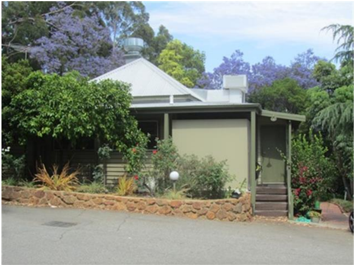
East elevation, (2015) (Photo taken by Shire of Mundaring)
