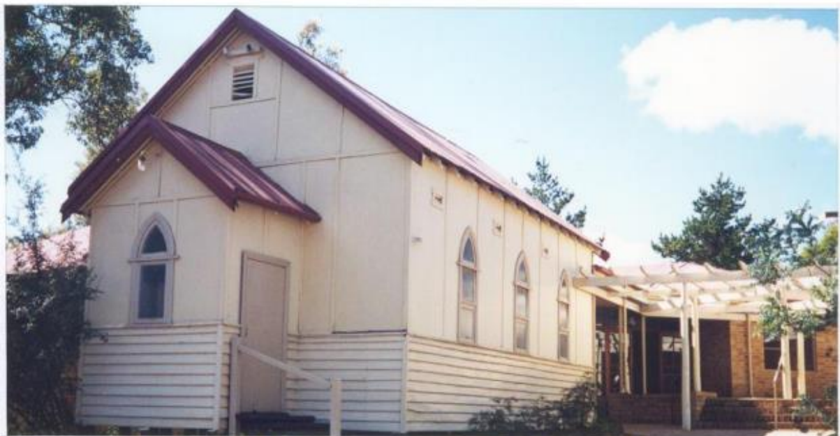
Front, west elevation of original building, August 1995 Bruce Callow & Associates Pty Ltd
