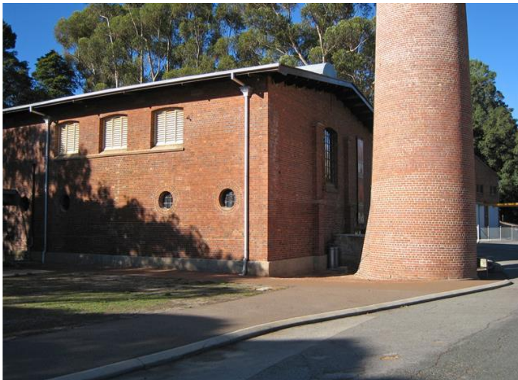
No.1 Pumping Station 2011
