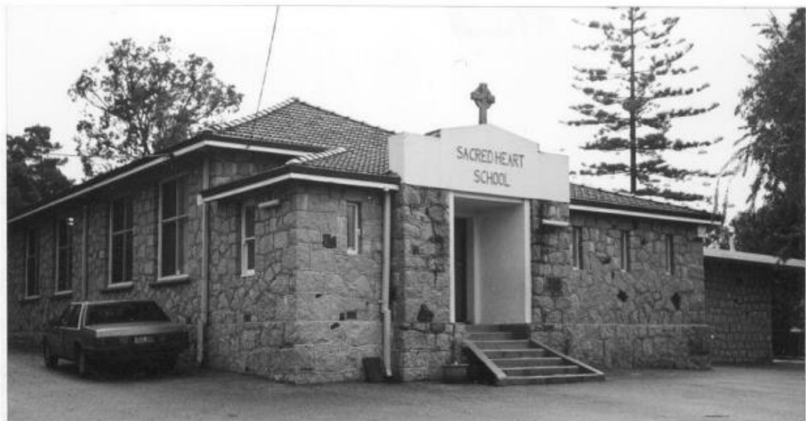
Top: Church - east elevation; Below: School elevation East August 1995 (Source: Bruce Callow and Associates Pty Ltd)
