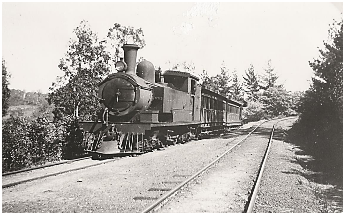
Mundaring Weir railway line (date unknown). (Source: Rail Heritage WA, P00603)
