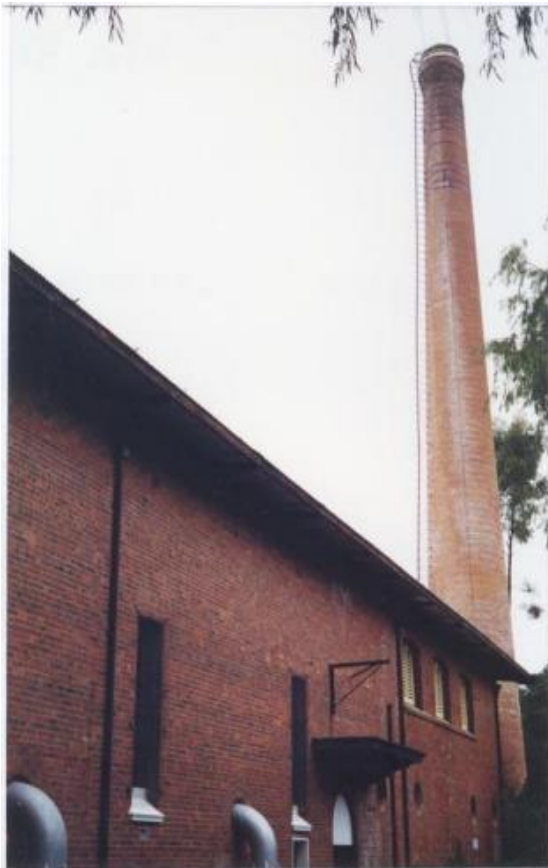
View of west wall and chimney, August 1995
