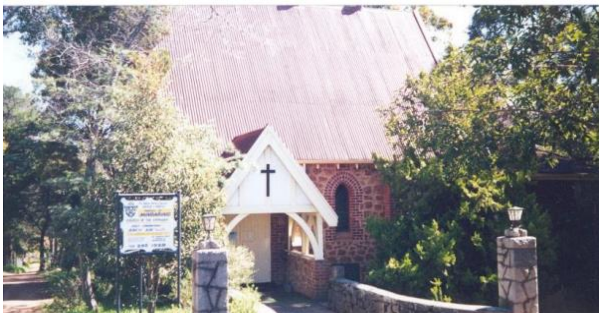
View of the church entry porch from Mann Street, August 1995 (Source: Bruce Callow and Associates Pty Ltd)
