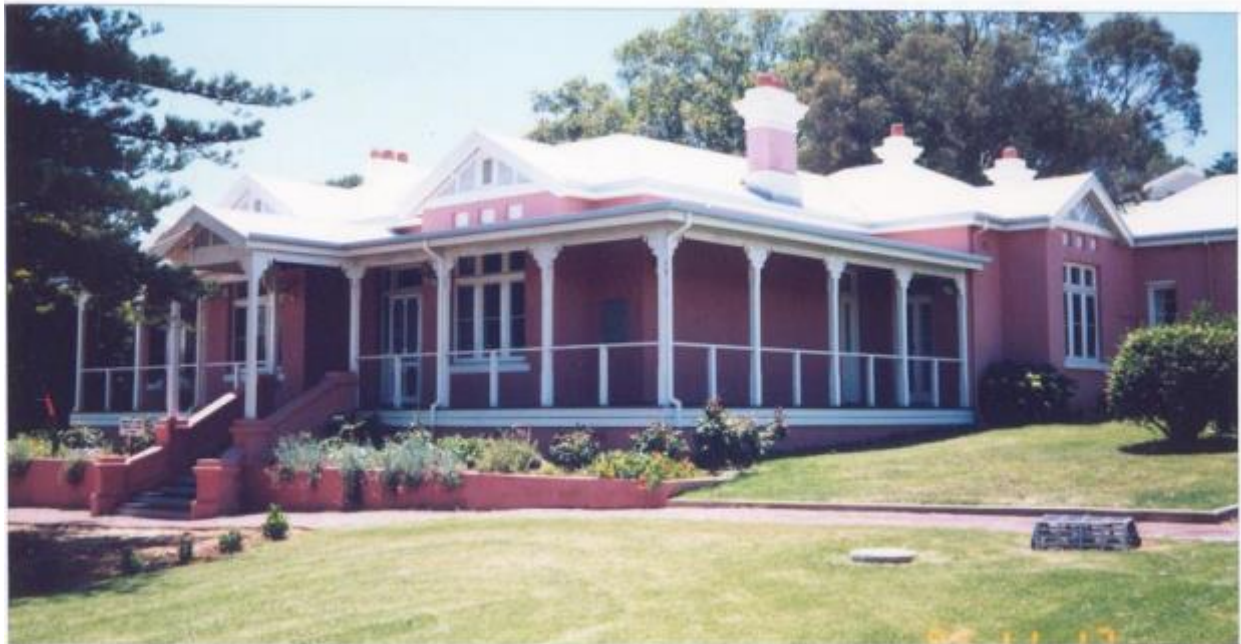
Original residence, south elevation, November 1995 (Source: Bruce Callow and Associates Pty Ltd)
