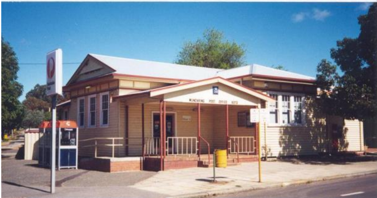
Mundaring Post office viewed from the north-east, August 1995 (Source: Bruce Callow and Associates Pty Ltd)
