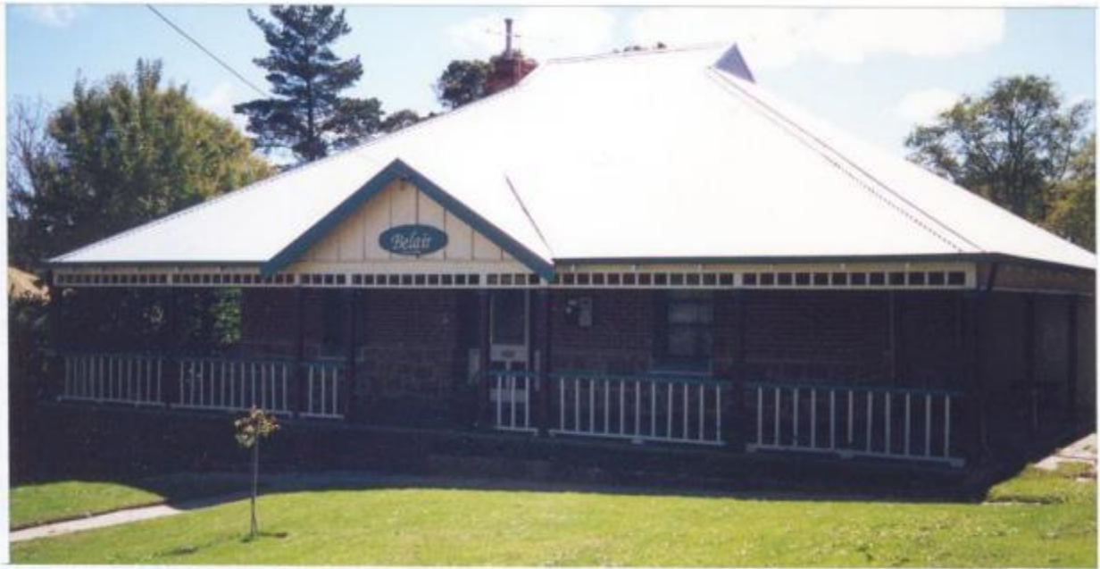
View from south-east, August 1995 (Source: Bruce Callow and Associates Pty Ltd)
