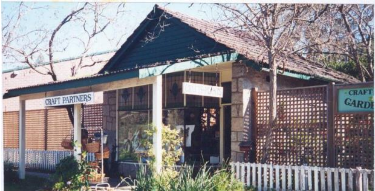
Front, south elevation, August 1995 (Source: Bruce Callow and Associates Pty Ltd)
