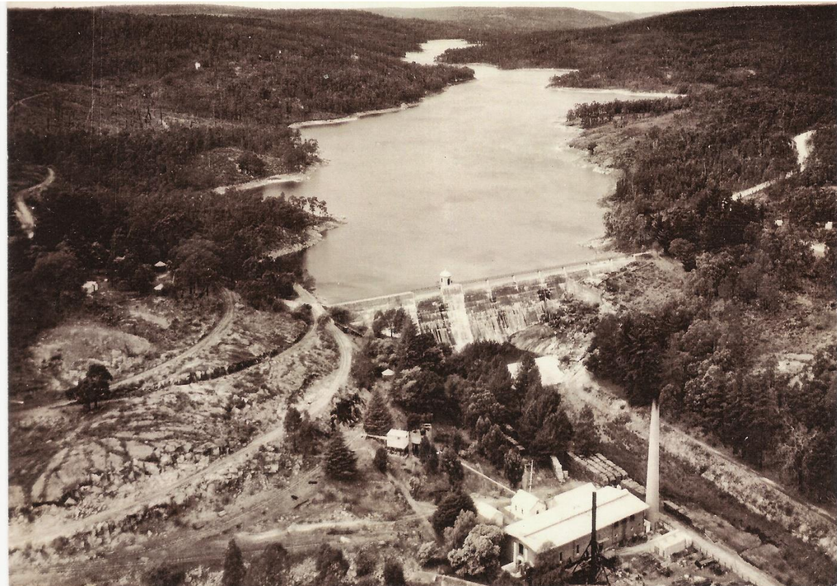
Mundaring Weir and pumping station no.1, aerial view taken from a RAAF aircraft (Source: Rail Heritage WA, P00590)
