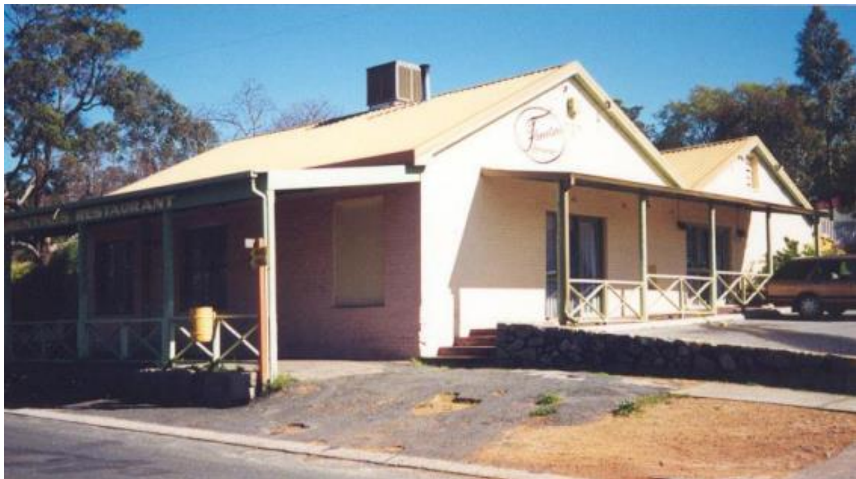
South and east elevation; former loading bay door, August 1995 (Source: Bruce Callow and Associates Pty Ltd)
