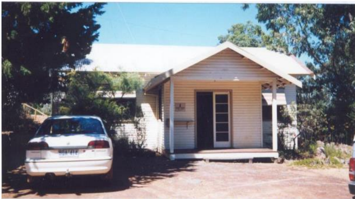
CALM Headquarters 1996 (Source: Bruce Callow and Associates Pty Ltd)
