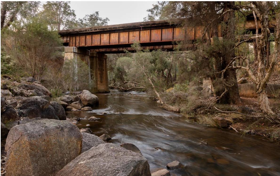
Railway Bridge in John Forrest National Park, 2023 (Source: Shire of Mundaring)
